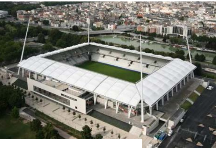
Stade de Reims, whose roof design allows light to reach the pitch
